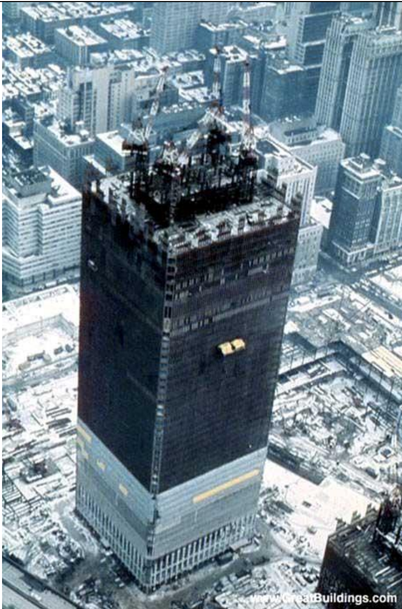
Figure 2. Construction of WTC1 (center of photo) began before WTC2 (lower right corner). The internal structures act as cross bracing.
